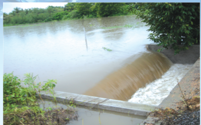
Plate 2. Recharge Basin Structure functioning during storm
