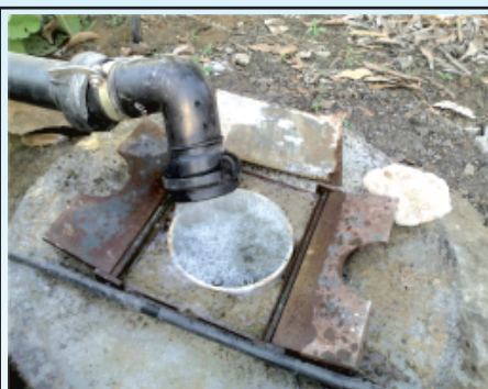
Plate 4. Tube well recharging at full recharge head condition
