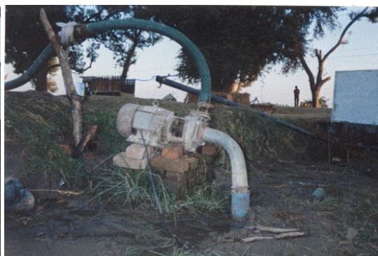
Firm foundation of the pump-rectified by the centre
