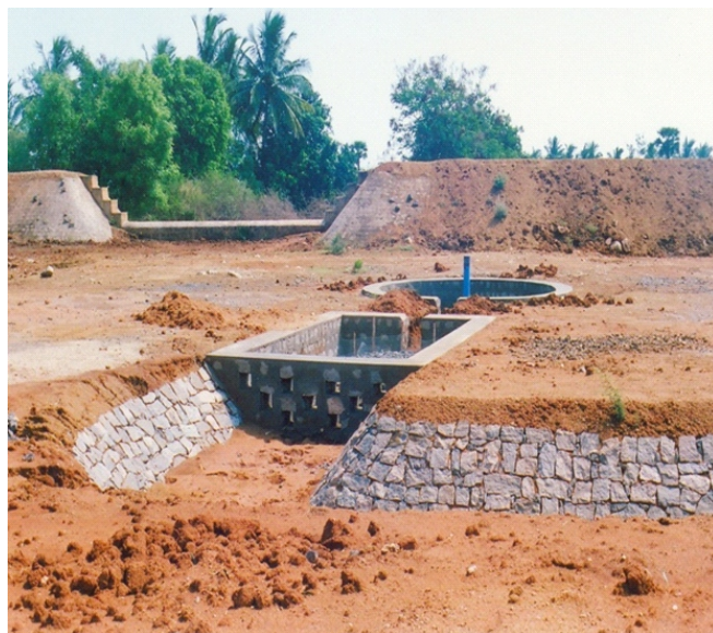
View of recharge borewell within percolation tank
