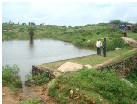
Low cost rainwater harvesting structure
