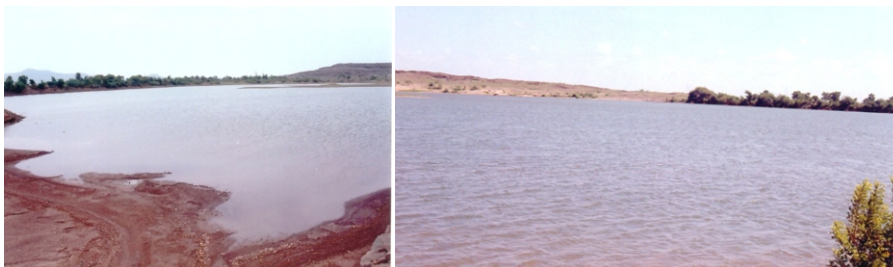
View of the percolation tanks
