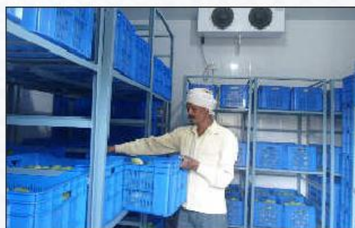
Fig. 11. Unripe mangos stored in solar powered cold storage
