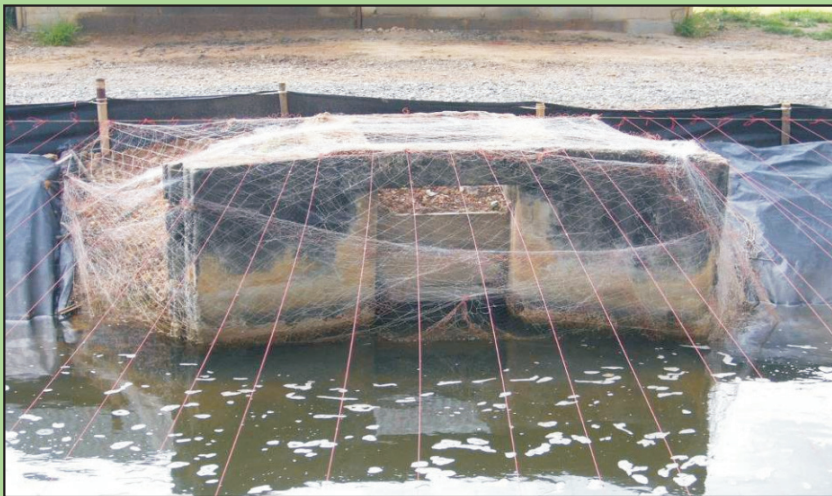
Fencing near sluice gate
