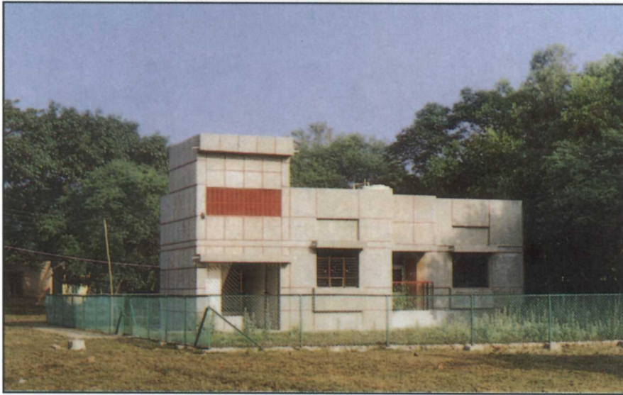
The newly constructed Type IV Staff quarters, at Kakdwip Research Centre of CIBA, Kakdwip, West Bengal.
