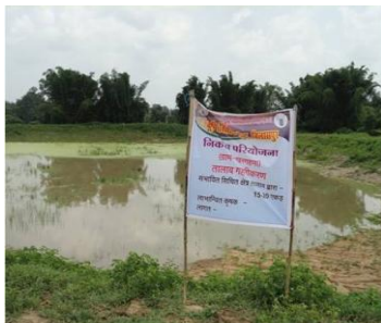
Rainwater harvesting structure
