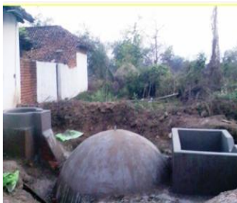
Construction of Biogas unit at Farmers field
