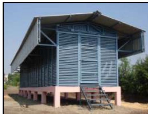
Fig 3. Side and bottom ventilated double row storage structure
