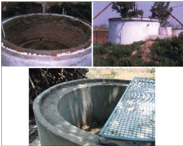
Insulated biogas plant
