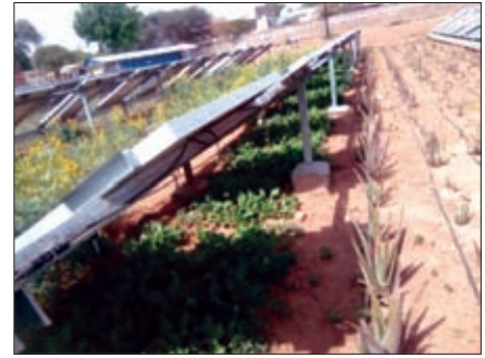
Fig. 3. Cultivation of spinach below photovoltaic module in agri-voltaic system
