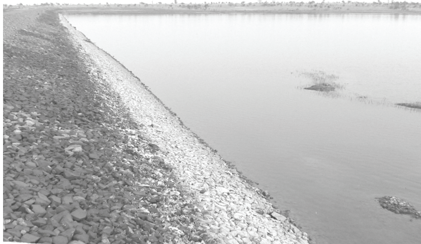
Photo 2 A big earthen checkdam constructed with labour contribution of beneficiary farmers for rain water harvesting to irrigate crop in Dharmapur watershed cluster of Vidarbha region of Maharashtra, India
