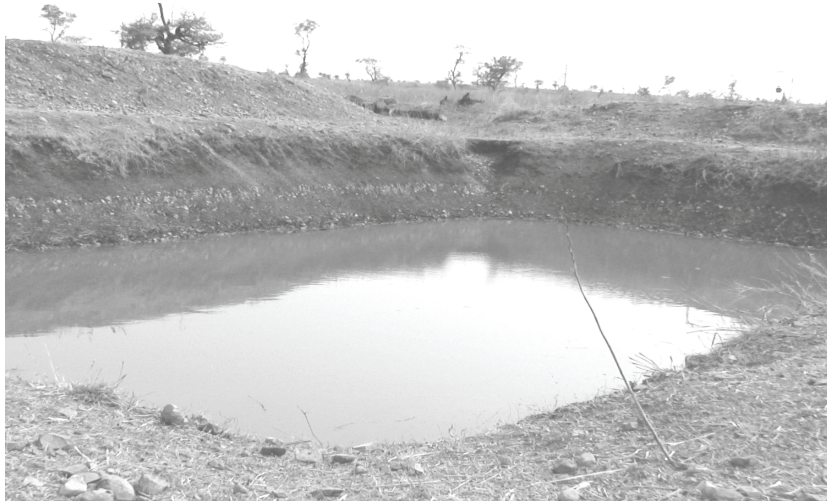
Photo 3 A farm pond in the field of a farmer for rain water harvesting to irrigate crop in waterscarcity conditions in Dharmapur watershed cluster of Vidarbha region of Maharashtra, India
