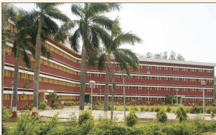
Modular laboratory building
