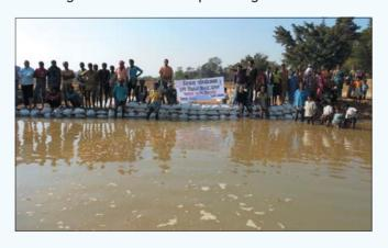
minimal cost. The temporary sand-bag check dam helped in impounding large quality of water for its use during post-kharif and entire rabi.
