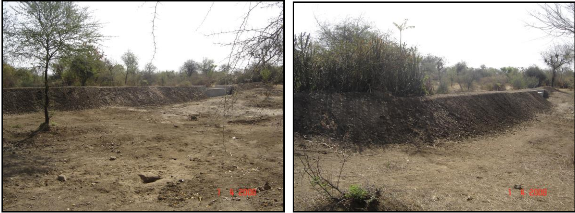
Fig. 2: Earthen water harvesting structure constructed in the study area
