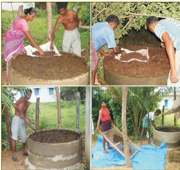
Figure 22 : Household level vermicomposting units at Tummalacheruve cluster in Khammam Dist.
