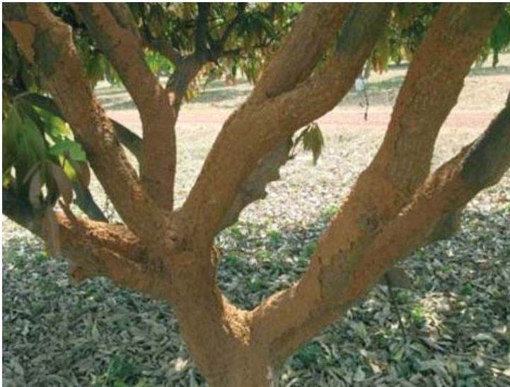
Tree trunk and branches infested with termites
