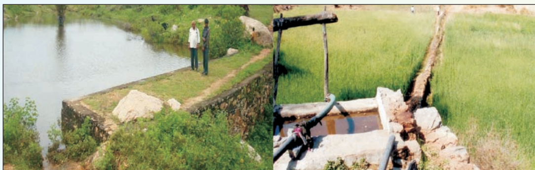
Effect of Dry Stone Masonry Pond on Groundwater Recharging of Open Well
