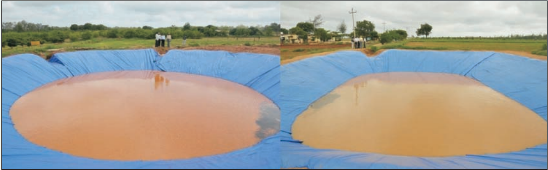
Water harvesting ponds (3 ha catchment-left) and 4 ha catchment (right) at CRIDA farm helped in life saving irrigation of crop in deficit rainfall year (2011)
