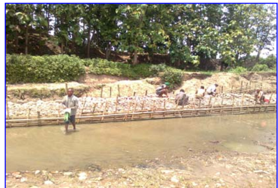
Construction of diversion channel in Dimapur, Nagland
