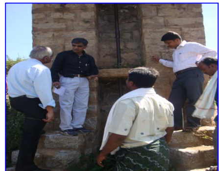
At village tank where sluice gate is repaired
