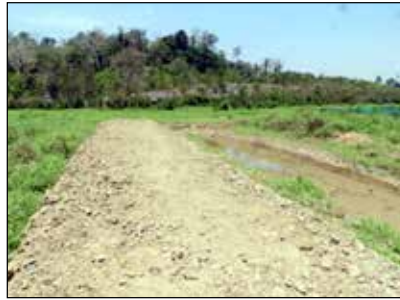
Plate 197: Road construction by MGNREGA
