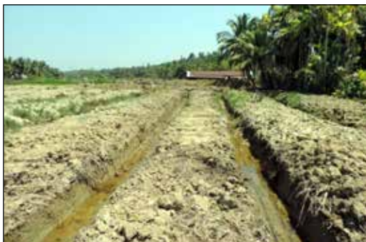
Progress of BBFS excavation at Kausalya Nagar
