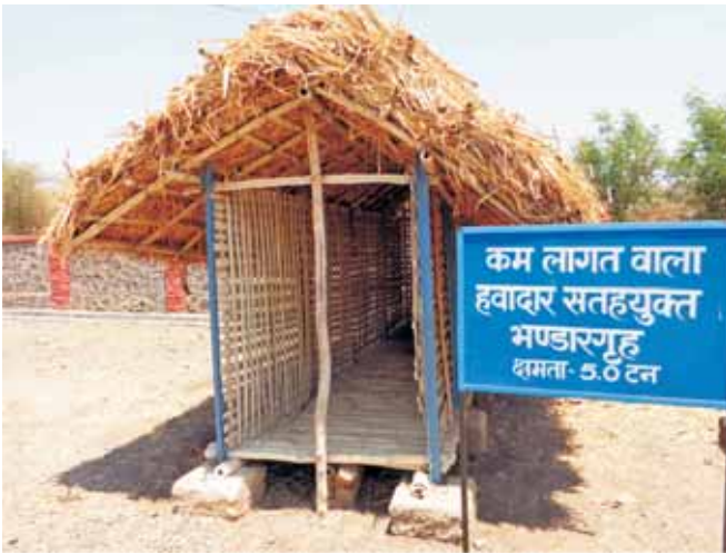
Low-volume low-cost onion storage structure
