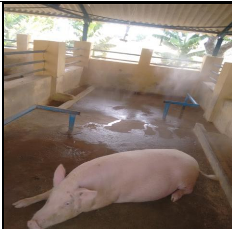
Installed foggers in the pig sheds
