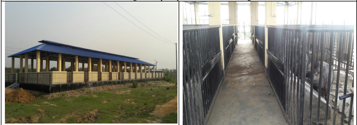
Newly established pig shed
