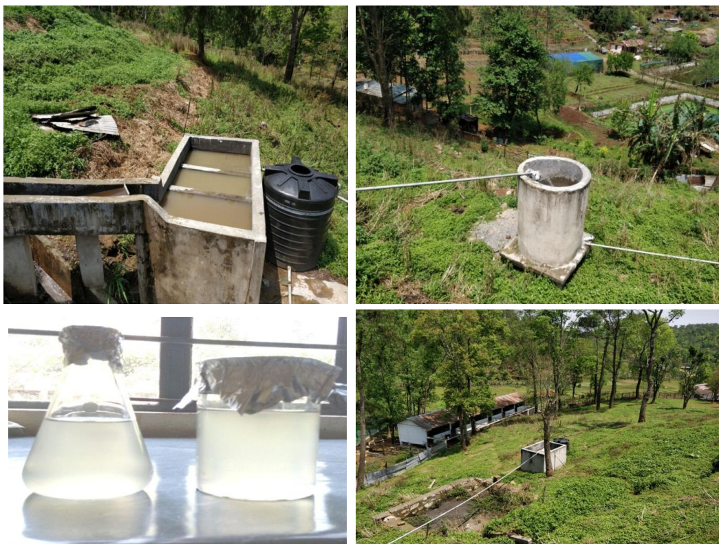
Pig-shed-wash water recycle unit through physical filtration technique
