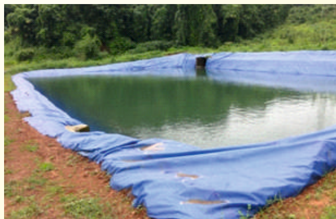
Rain water harvesting pond
