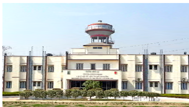
The capacity of the 'Visiting Scientists Home' has been increased with the completion of the vertical extension work
