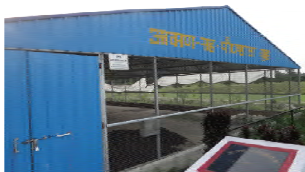
Screen House cum Potting Shed for multiplication of litchi planting materials
