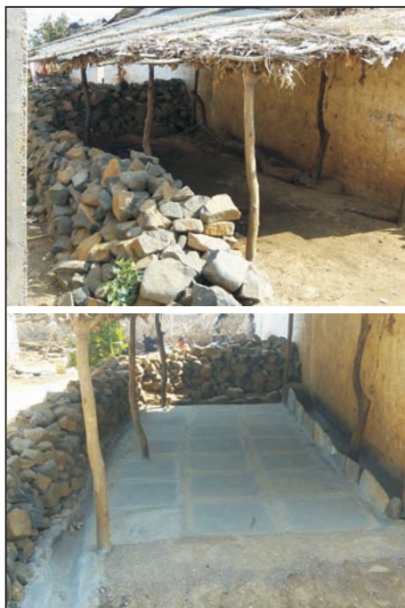
Cattle shed before (top) and after (bottom) intervention
