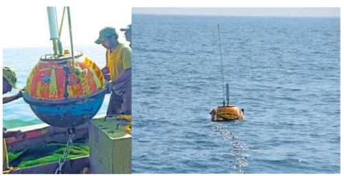
Photograph showing wave rider buoy installation
