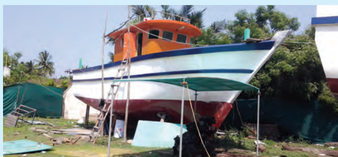
The 13.7 m L OA FRP Tuna fishing boat under construction at Cuddalore for Andamans
