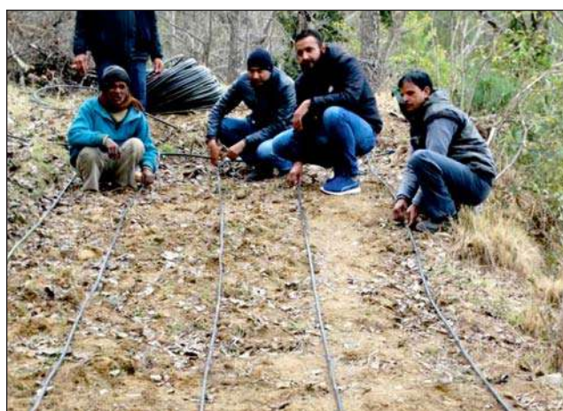
Installation of drip irrigation system in Salla Rautela village
