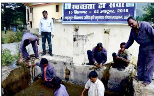
Cleaning of water tanks at Hawalbagh campus
