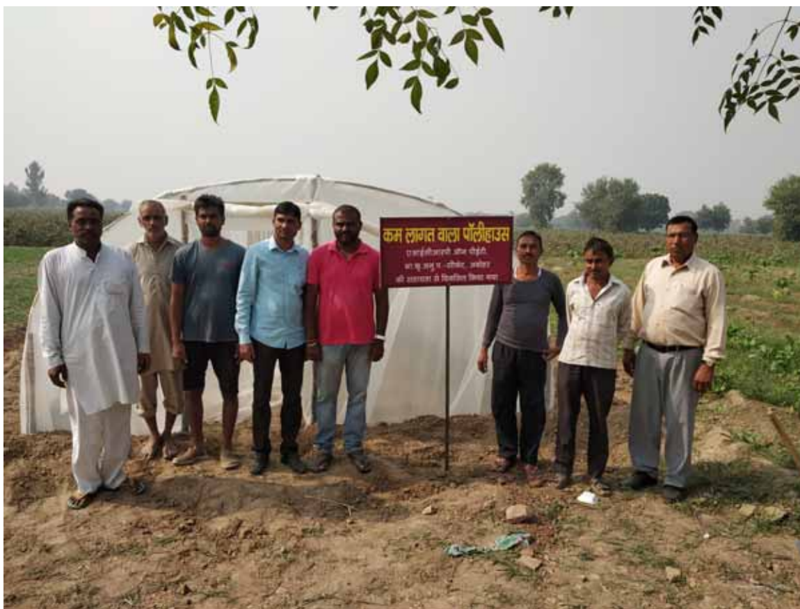
AICRP on PET, ICAR-CIPHET Abohar constructed four low-cost polyhouse structures (floor area 60 m 2 ) at farmers' fields in the village of Amarpura and Kala Tibba
