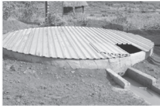
Fig. 5. Underground storage structures
