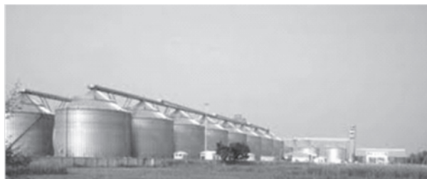
Fig. 7. Typical view of the grain storage structure
