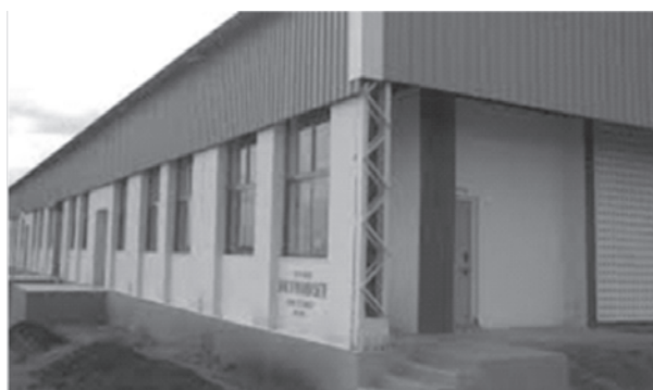
Fig. 8. Typical Bulk Cold storage structure for fruits
