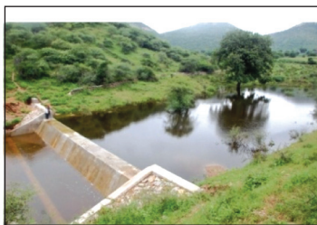
Masonry check dam at Karget
