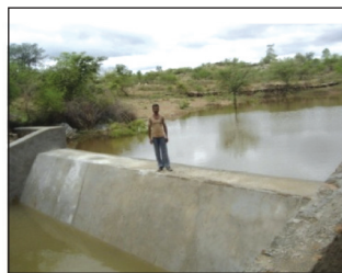
Masonry check dam at Shishvi
