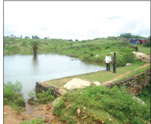
Low cost dry stone masonry structure constructed at Shishvi village
