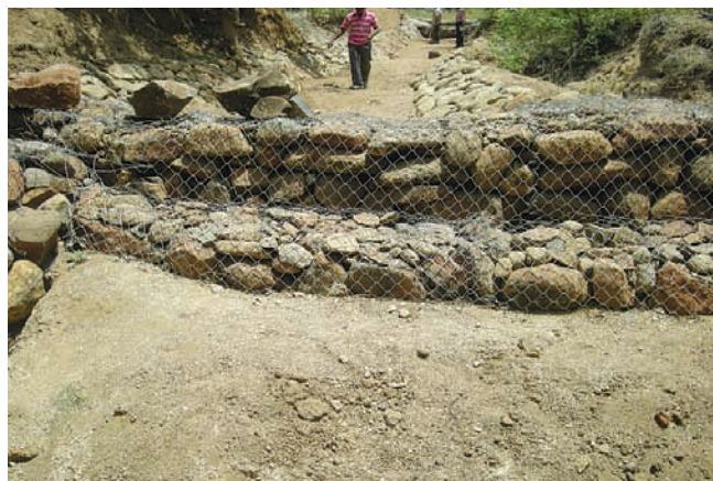
Two-stepped gabion structure
