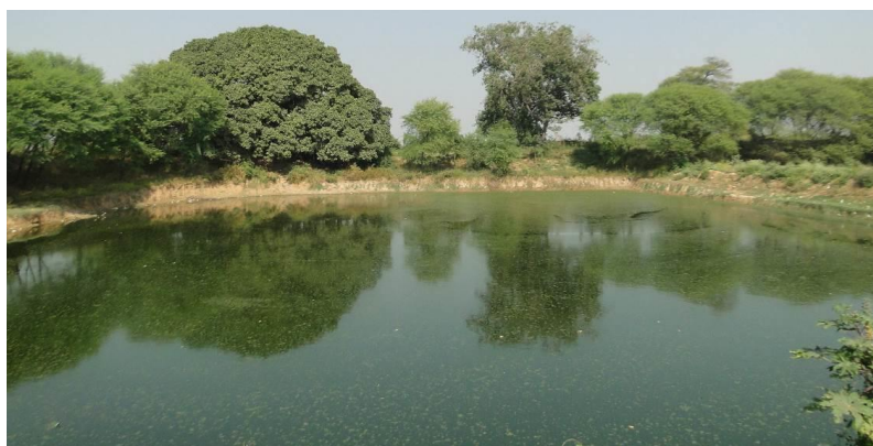
Renovated water harvesting structure – village Nainwan
