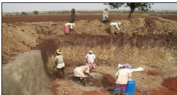
Farm pond lining with red soil and cement (6:1 ratio)
