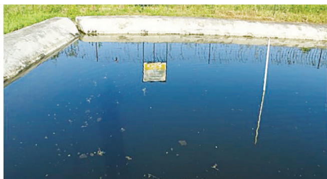
Cement concrete lined farm pond with harvested rainwater
