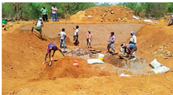
Mixing of red soil + cement (6:1) as lining material
