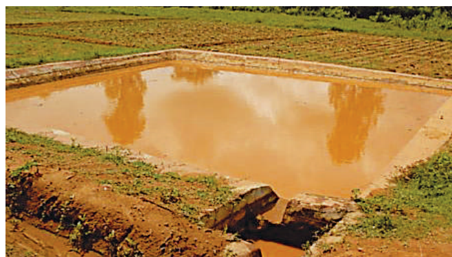
Lined farm pond with harvested runoff
