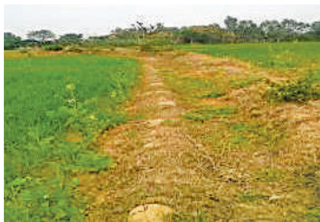
Stone pitching on bunds
