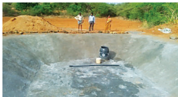
Farm pond after lining
