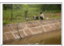
Fig-5 Lifting of water through portable pump set and irrigation to crops 130 m away from pond
