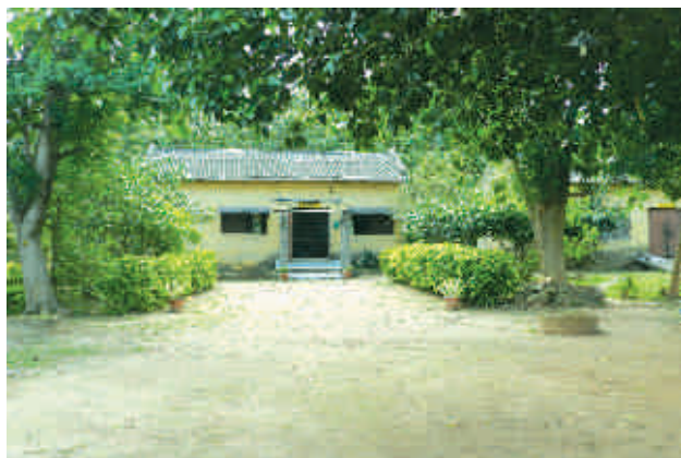
Main building of KVK Cuttack
