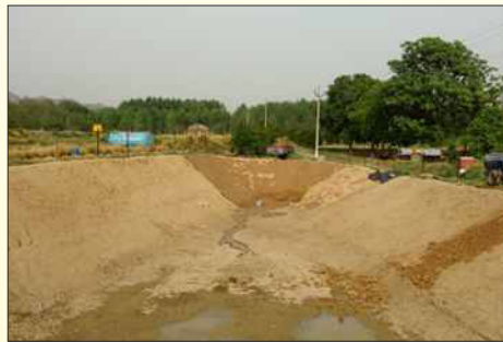
Construction of farm pond
