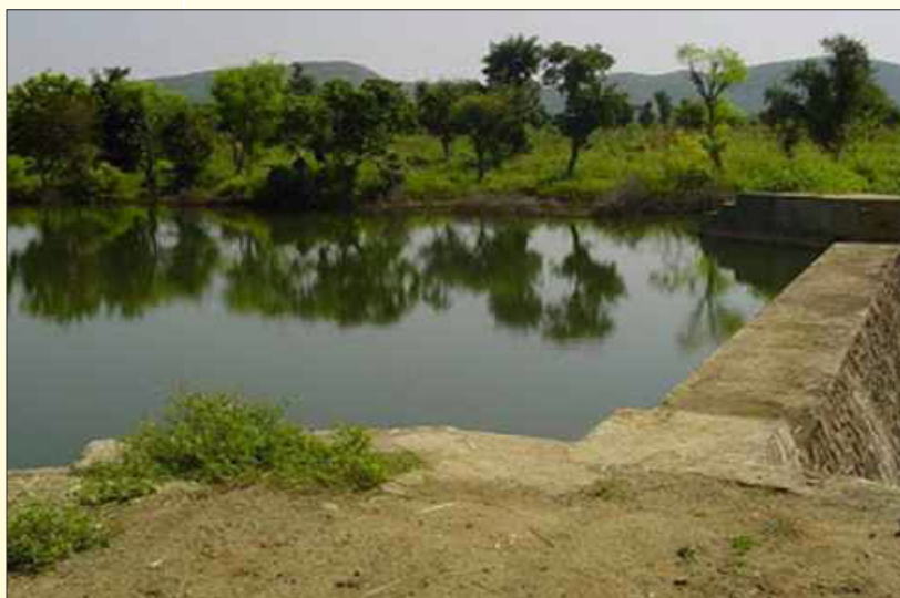
Masonry check dam
