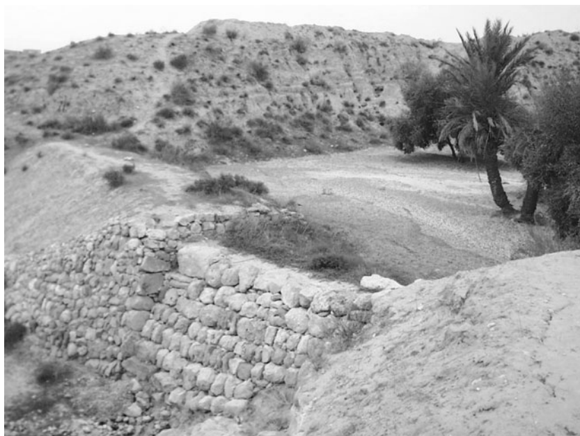
Fig. 9.3. Jessours are widely practised in Tunisia for water harvesting.
