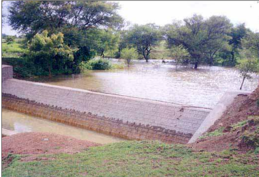
Figure 4. Water stored in check dam built across the stream channel (ex-situ management); Photo: Kothapally watershed.
