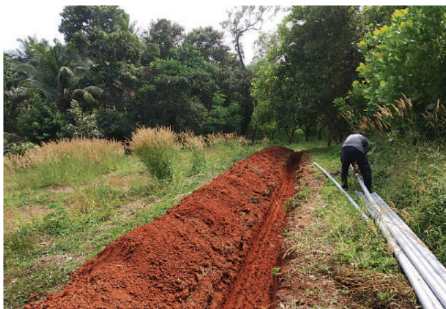
Fig. 12. Laying the main line of the drip system
