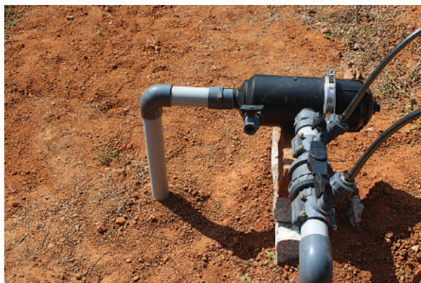
Fig. 14. Disc filter
