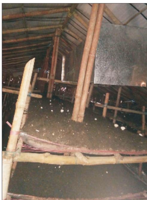
Internal View of Mushroom house fitted with Duct System
