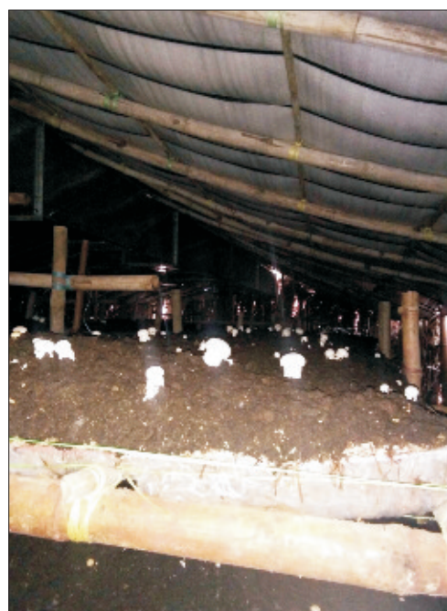
Insulated roof of Mushroom house
