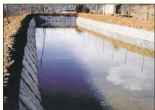
LDPE-lined tank (280 m 3 size) constructed at Darim village for micro-irrigation system
