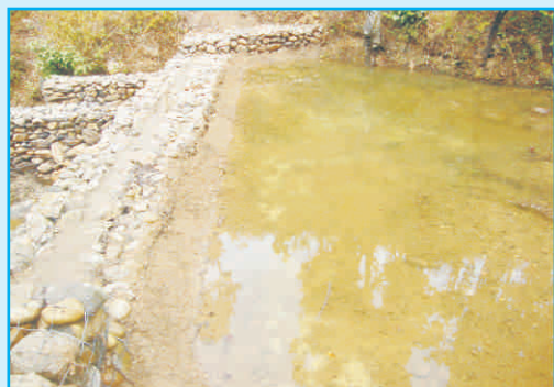
Low-cost HDPE Sheet Embedded Gabion Checkdam for Water Harvesting
