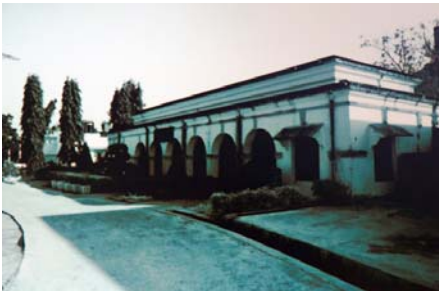
Old Building of CRRI
