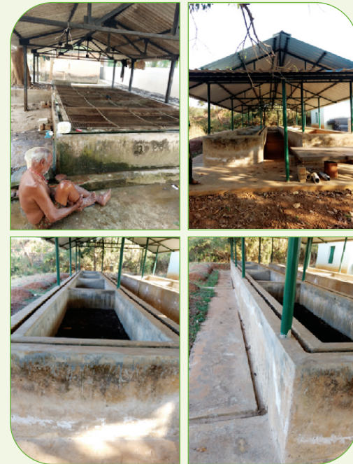
Fig.2 Permanent Protected Vermicomposting units with drainage outlet
