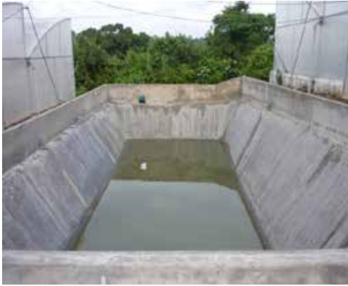
(c) Finished lined tank
