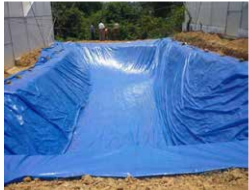
(b) Laying of Silpaulin
