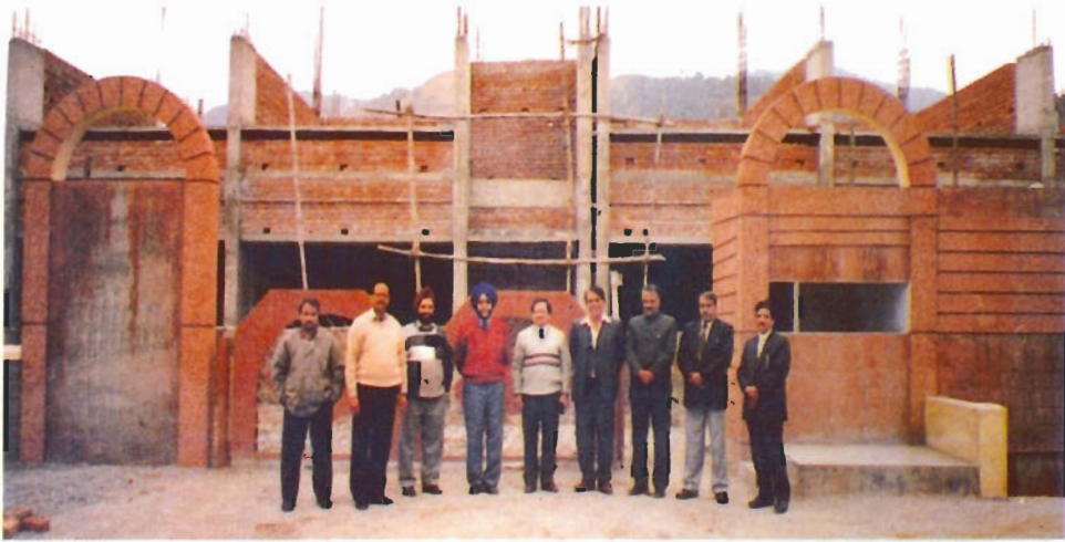
Management Committee members visiting the NRCCWF complex (under construction)
