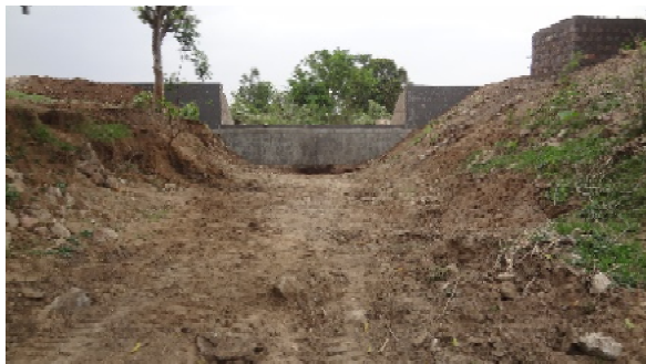
Drop structure and gauging station in Bachhauni village of Watershed
