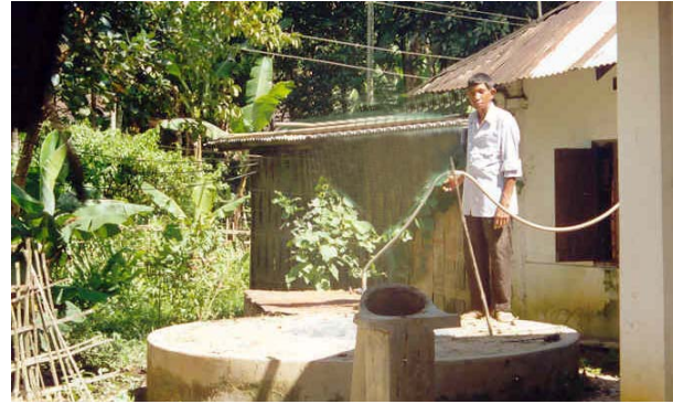
Biogas plant in a village near Jorhat (Assam)
