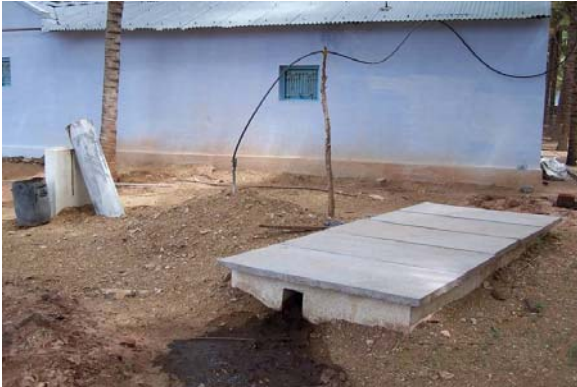
Solid state BGP of 3 m 3 at a farmer's at village Periapatti (TN)
