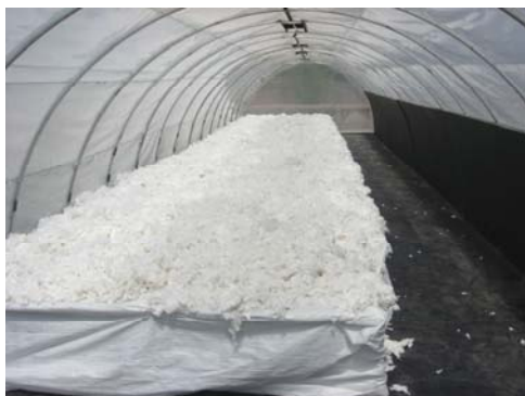
Solar tunnel dryer installed at M/s Cotton Products India, Udaipur
