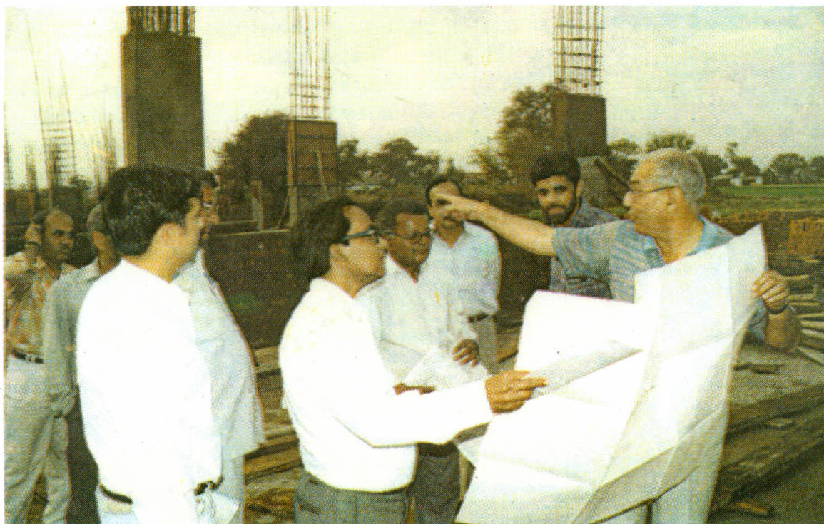
Fig.-13: Centre's Management Committee surveying the progress of building construction.
