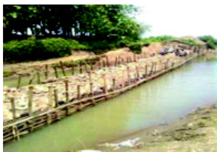
Fig 9 Diversion of irrigation channel under NICRA at Dhanshirpar village, Dimapur
