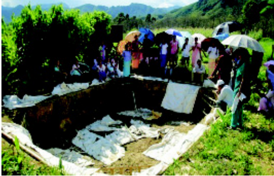
Fig 9 Construction process of Jalkund
